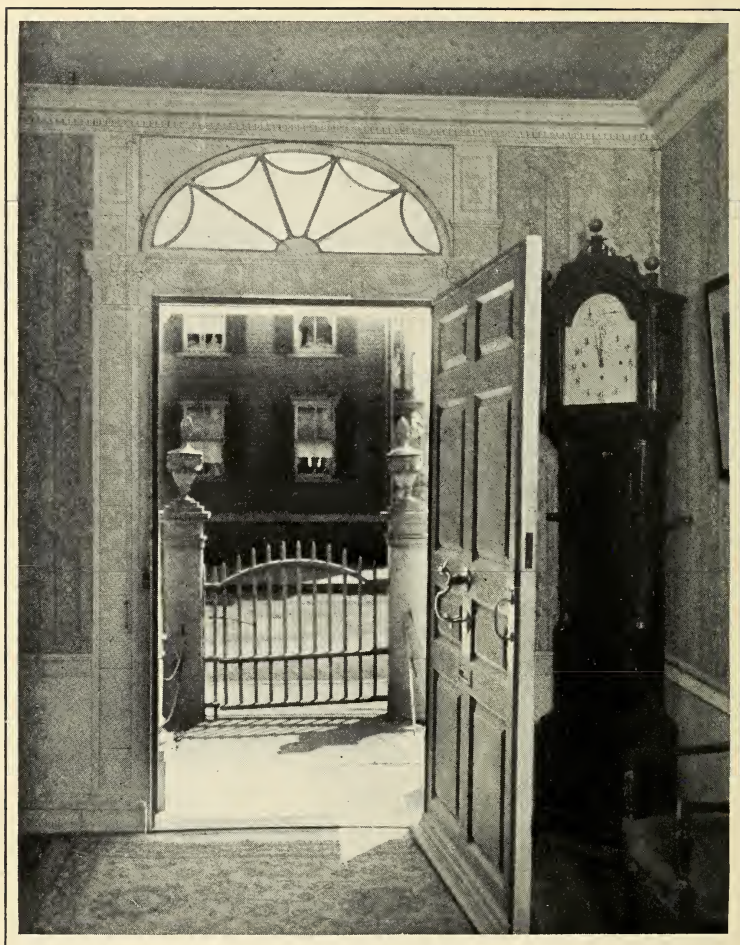
Hall in the Nichols house, Salem, designed by McIntire. The picture includes the original carved gate-posts as well as a bit of the fine woodwork.
